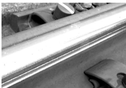
Photo 2: Wear on inside edge of outside rail on curve (JR East)
