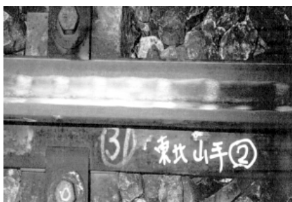
Photo 1: Corrugation wear along rolling surface of rail head (JR East)
