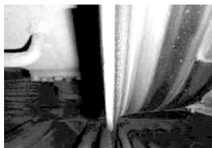
Photo 3: Rectangular wear at inside arc profile of wheel flange (JR East)
