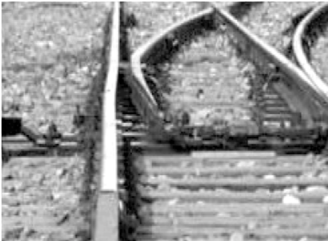
Photo 8: Deformed main rail next to switch tongue rail
