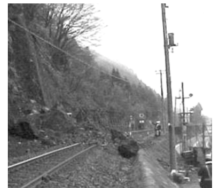
Rockfall blocking track
