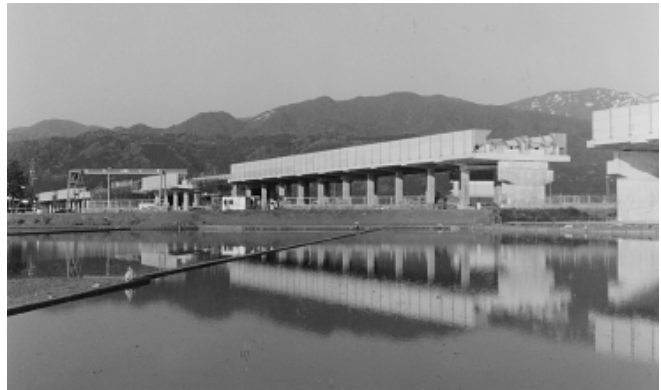
Construction of elevated section of Hokuriku Shinkansen in Toyama Prefecture due for completion in 2012 (Author)
