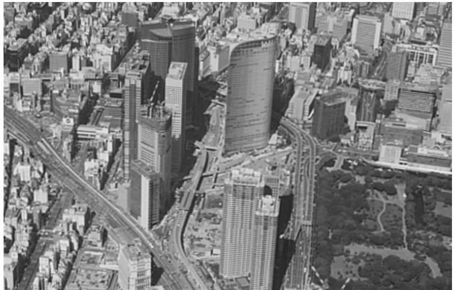
Aerial view of redeveloped Shiodome site in September 2002
