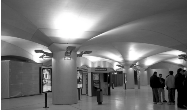
Transfer floor at Bibliothèque François Mitterrand Station
