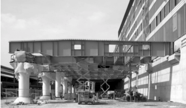
Construction site of Austerlitz Station
