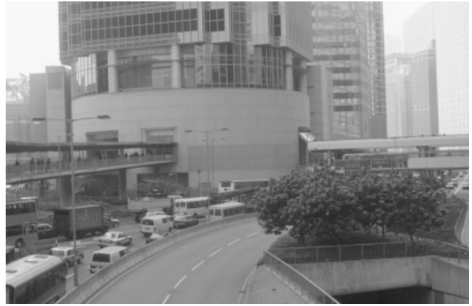
Podium for skyscraper at Hong Kong Station serving as interconnecting concourse for pedestrian traffic (Author)
