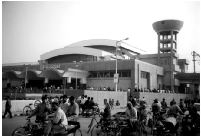
Shahdara Station of Delhi Metro Line 1
