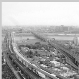
Tsukuba Express Line under construction at Kita Senju, Tokyo, crossing Arakawa River alongside TRTA's Chiyoda subway (far left), JR East's Joban Line (left) and Tobu Railway's quadruple Isezaki Line (right). (JRCC, Tokyo Regional Bureau)
