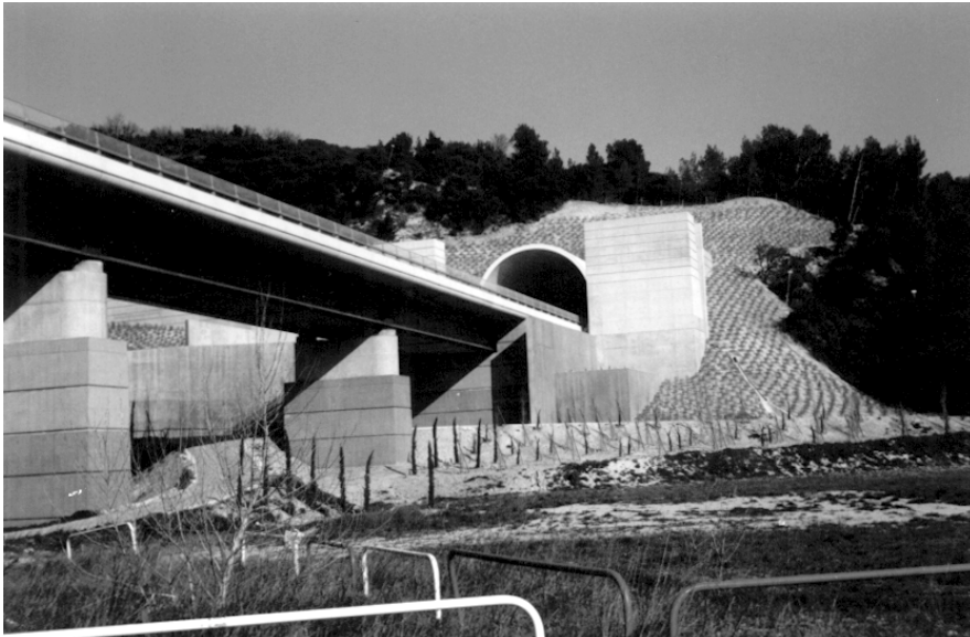
Management of and investment in infrastructure is the responsibility of RFF. (Author)
