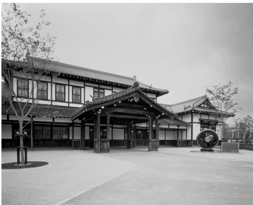
The former Nijo Station and now part of USLM
