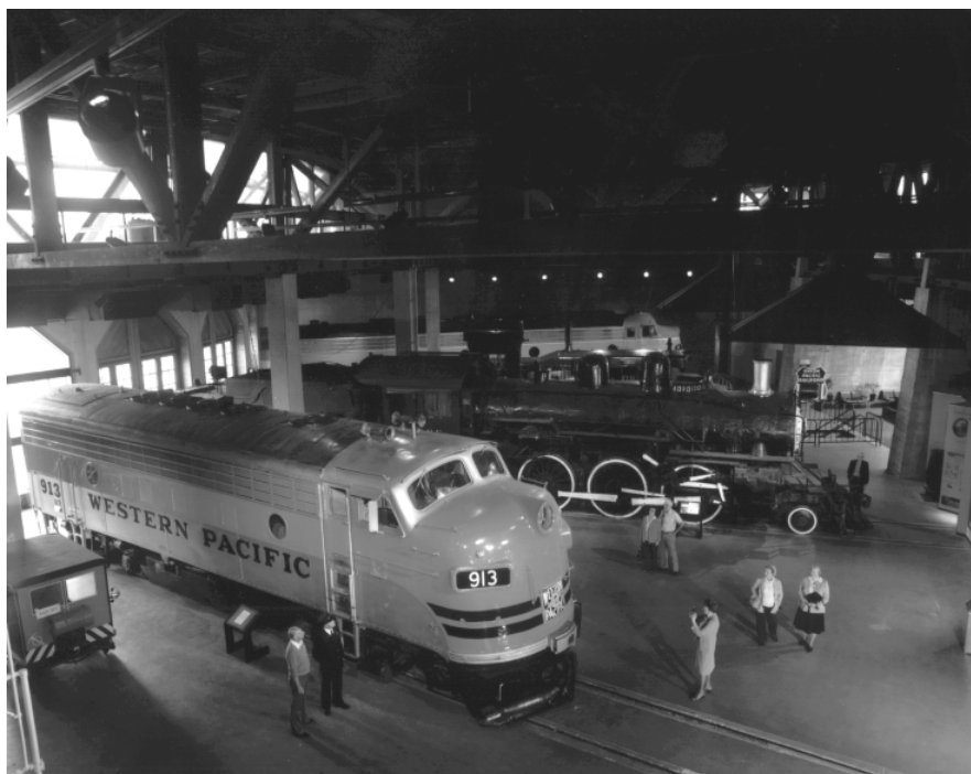
Inside the roundhouse area of CSRM, guests are invited to step aboard several exhibits including a Pullman-style sleeping car complete with night-time lighting, motion and sounds, and a dining car filled with railroad china. (CSRM)
