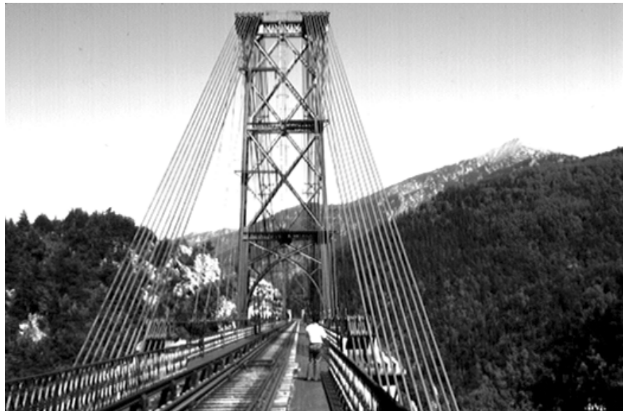
SNCF's meter-gauge Cerdagne Line in the Pyrénées with famous suspension bridge designed by Albert Giscard. (EJRCE)
