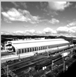
Hachinohe Station at northern end of Tohoku Shinkansen extension almost completed 1 year before its official opening in December 2002. A Tokyo- bound container express is seen at the front. (Transportation News)
