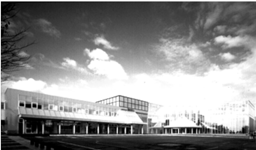
Yamagata Shinkansen terminus at Shinjo Station (The Association of Railway Architects)
