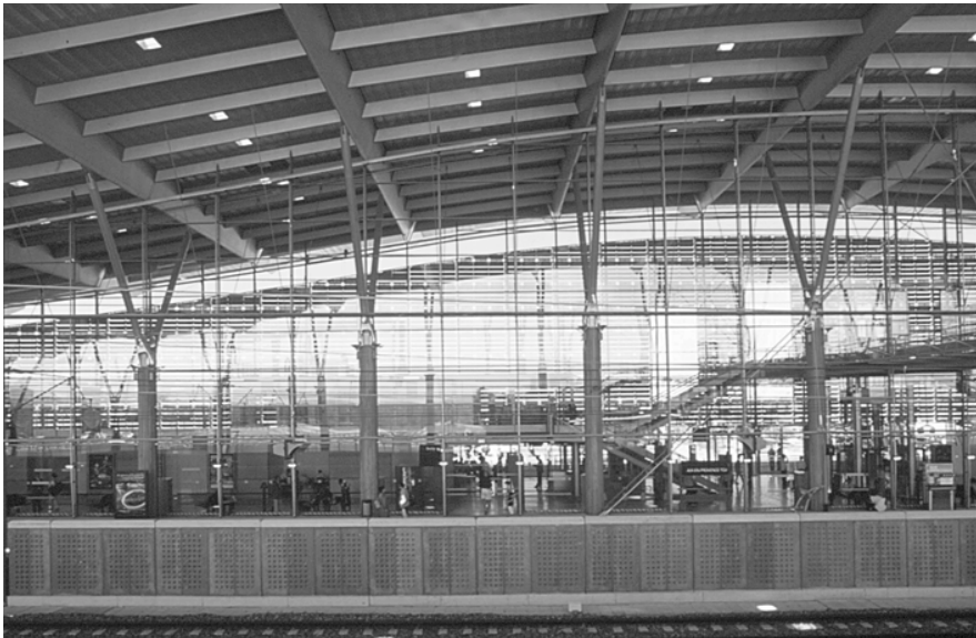
The tree-like pillars of Aix-en-Provence Station allow a great visual depth. (SNCF AP-AREP, M. Denancé)
