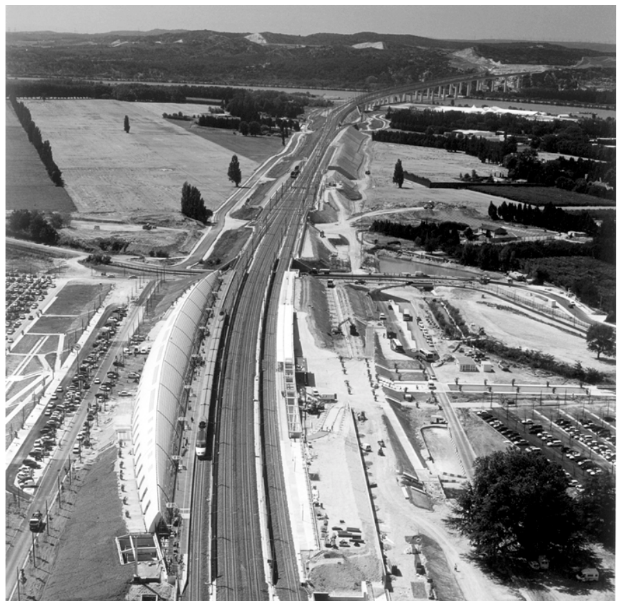
Avignon Station's descending pointed archway has the dual function of a station hall and a platform. (SNCF AP-AREP, P. Charpiot)
