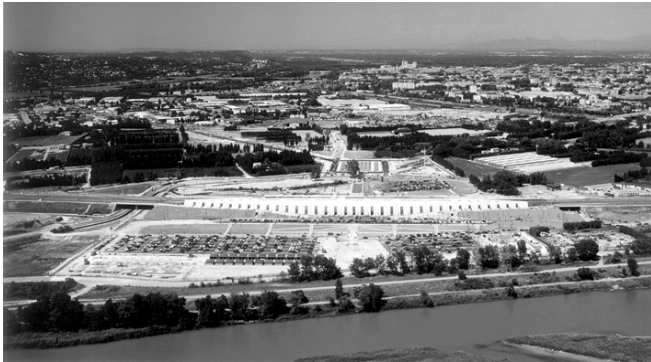
The slightly curved Avignon Station emerges between the River Durance and the city. (SNCF AP-AREP, P. Charpiot)
