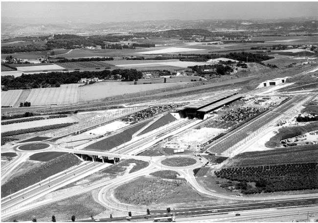
The train arriving at Valence Station, running through a cutting of the Drôme Plain
