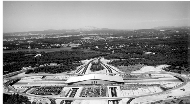
Aix-en-Provence Station forms a crossroads with a highway, creating a perfect connection between road and rail. (SNCF AP-AREP, P. Charpiot)
