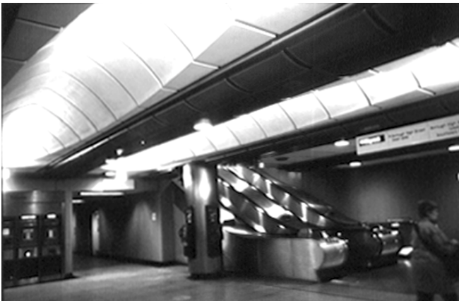
London Bridge Station
