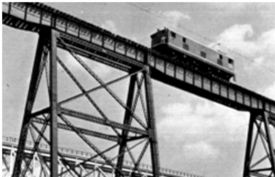
Class ED44 locomotive testing AC electrification on Senzan Line near Sendai in north Honshu (JNR Centennial Photo History)
