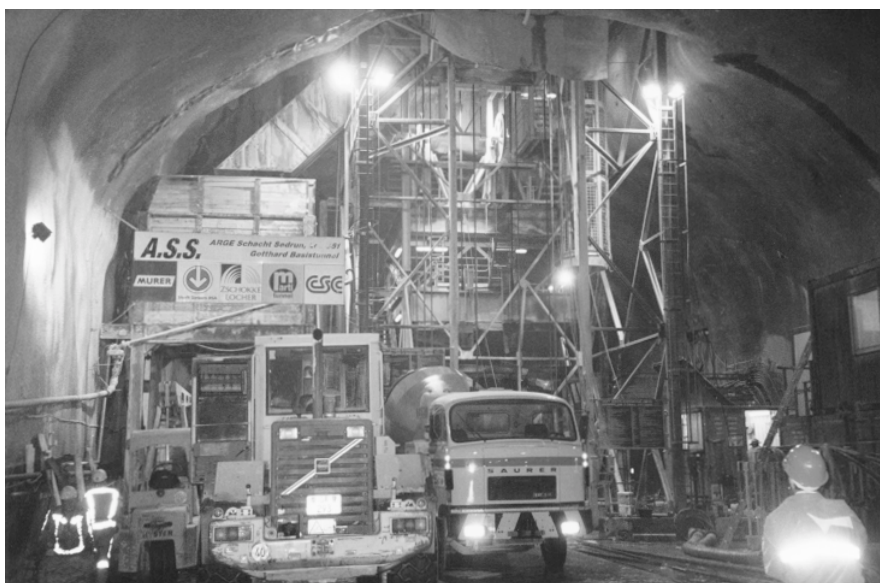
Vertical shaft at new St. Gotthard Tunnel
