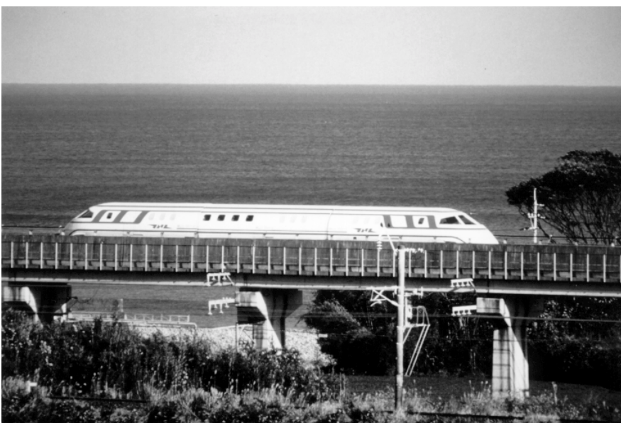
MLU001 Three-car train on Miyazaki Test Track
