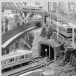
TRTA Marunouchi Line crossing River Kanda beneath JR East Ochanomizu Station where Sobu Line (yellow train in distance) branches off from Chuo Line (orange train) (EJRCF)
