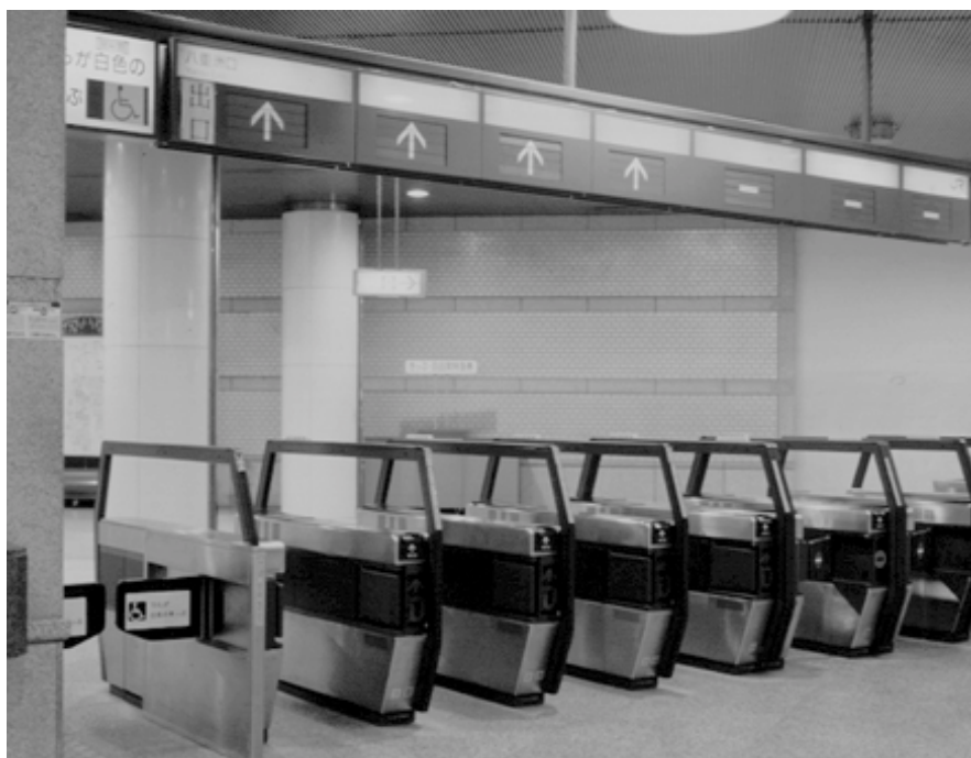
Latest magnetic automatic ticket gates
