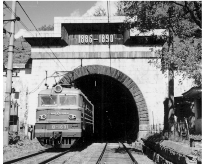
Tsipa Tunnel (4 km, 777 m above sea level)
