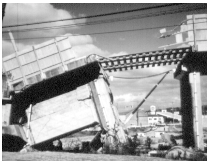
Viaduct collapsed during Great Hanshin Earthquake
