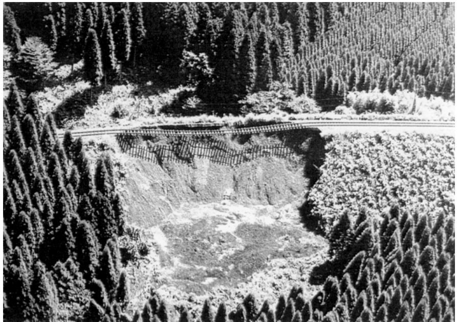
Embankment collapse caused by heavy rain
