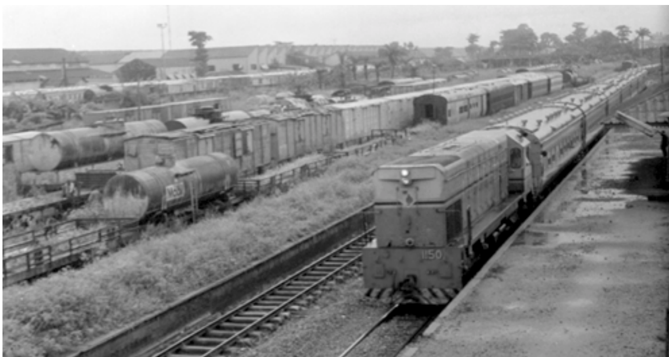
Large numbers of wagons abandoned in unmaintained yard at Ebute Metta Junction, Lagos
