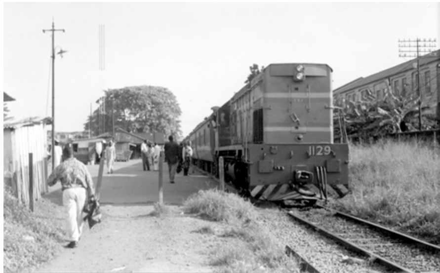
Poor state of tracks before rehabilitation
