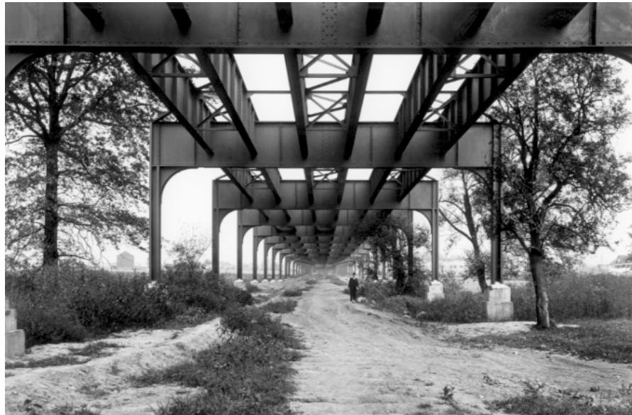
This is a photograph of the elevated portion of a new subway line to Queens being constructed under the Dual System plan of 1913. The date is 8 October 1914. This line starts at Times Square in Manhattan, crosses 41st and 42nd streets and then passes under the East River to Queens. When it opened to Corona in 1917, the services on the line were jointly operated by the Interborough Rapid Transit Company (IRT) and Brooklyn Rapid Transit Company (BRT). The line now terminates in Flushing. This view is looking east through what was then open land. This area was only about 5 km from the East River separating Queens from Manhattan. The main purpose of the Dual System was to open up new districts of New York for residential development.
