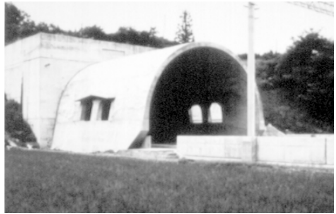
Concrete tunnel hood at the Daini-arikabe Tunnel (JR East)
