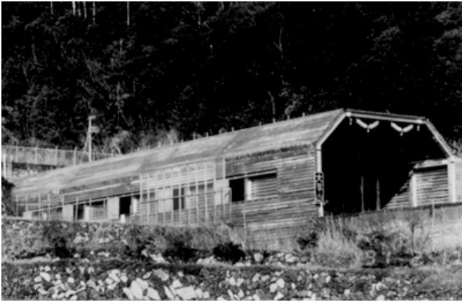
This hood at the entrance to Ohirayama Tunnel (6640m) on the San'yo Shinkansen is 49 meters long. If it had been constructed at the same time as the line, it would have been concrete. (JR West)
