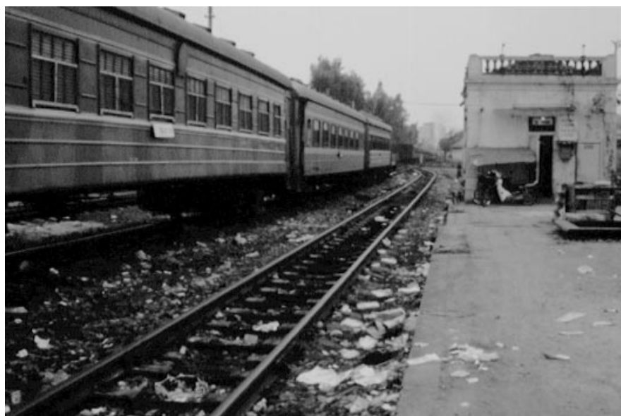
Littered track and rundown station buildings typify some of the modernization problems.
