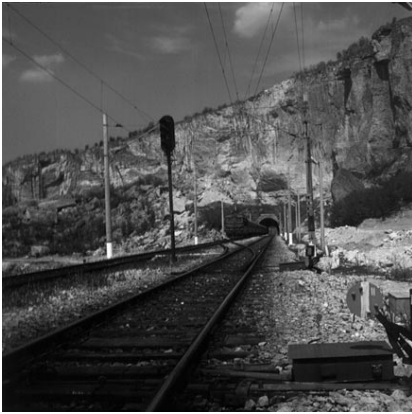
Portal of cross-border tunnel in B02 network (BDZ)
