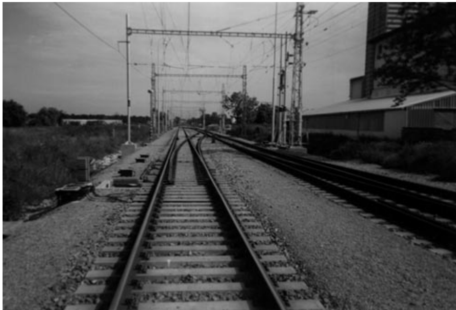
Reconstructed track on Brno–Breclav section of Crete Corridor IV
