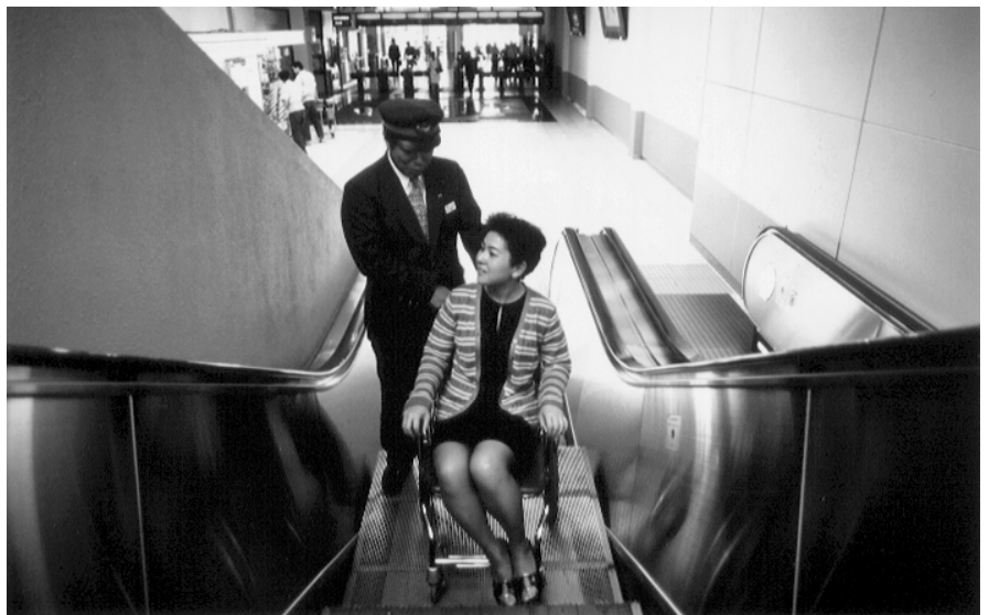
Wheelchair platform installed on escalator
