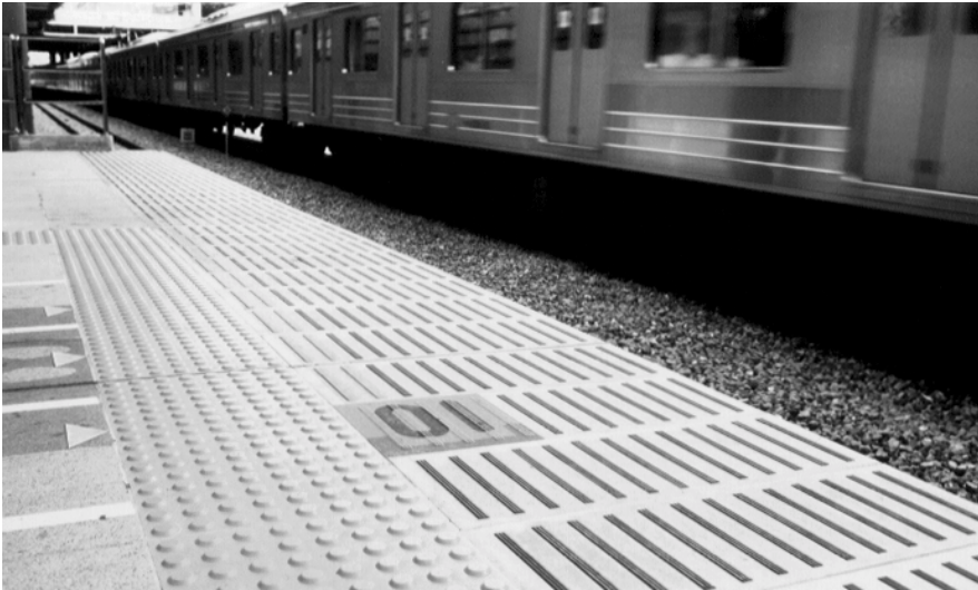
Tactile tiles on platforms guide and warn people with impaired vision of hazards.
