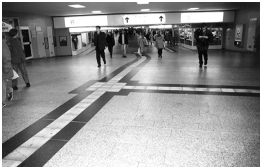
Duisburg railway station in Germany has tactile guideways to orientate people with vision impairments. (Author)
