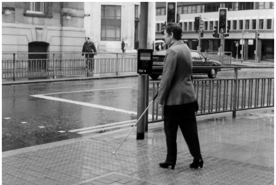
Tactile surfaces warn visually-impaired people of hazards (UK Department of the Environment, Transport and the Regions, DETR)
