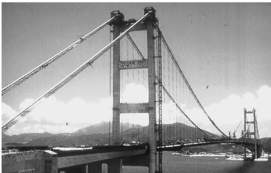
Tsing Ma Bridge in Lantau Link
