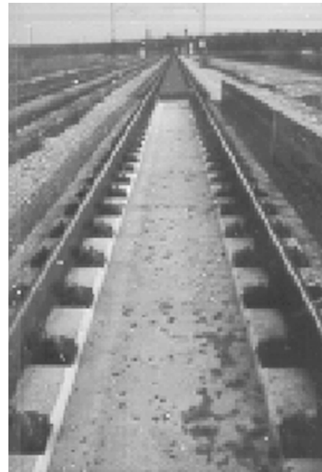
Slab track with ultra-low-acoustic barrier on high-speed test line between Karlsruhe and Mannheim (DB AG)
