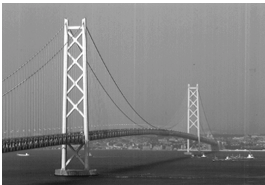
Centre span (1990 m) of recently opened Akashi Kaikyo Bridge linking Kobe and Awaji Island (Transportation News)
