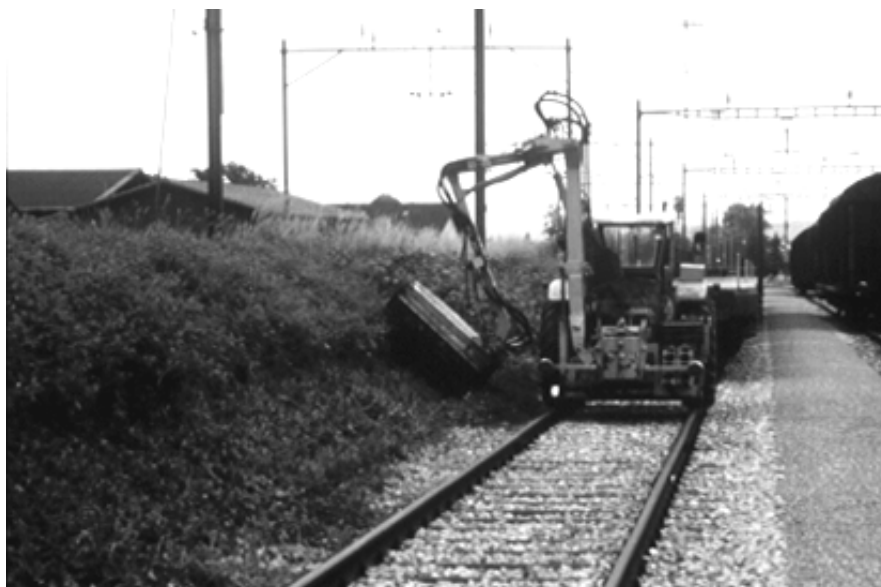
Maintaining greenery by mowing embankment
