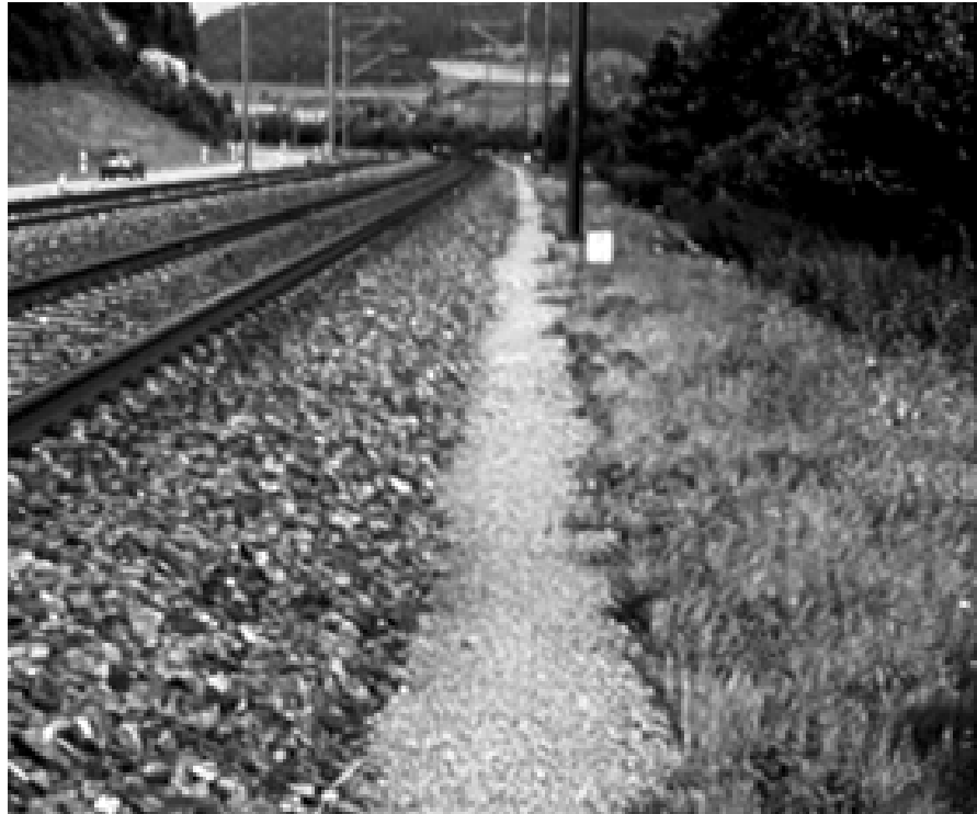
Concrete barrier to in-growth of plants
