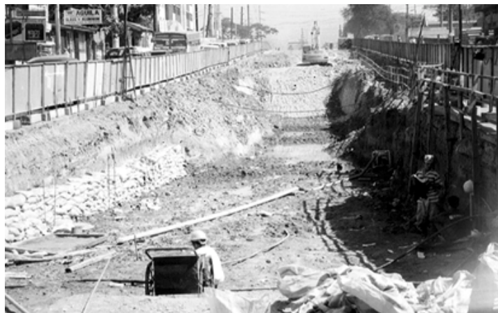
LRT Line 2 under construction
