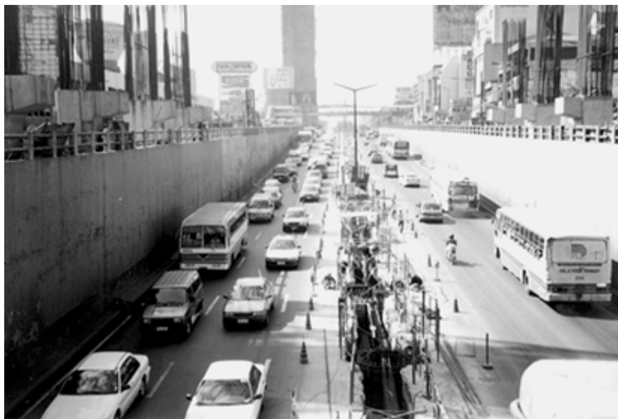
Looking south from Shaw Boulevard overpass on LRT Line 3 with part of EDSA straddled by station support columns (EDSA MRT Project)
