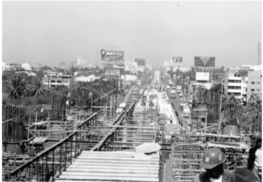
Workers preparing roof of Santolan Road Station on LRT Line 3
