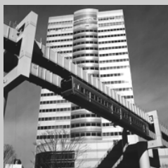
Suspended monorail with Chiba Monorail Station Building in background (Chiba Urban Monorail Co., Ltd.)
