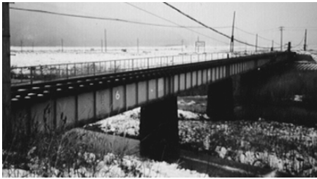
Plate girder bridge (RTRI)
