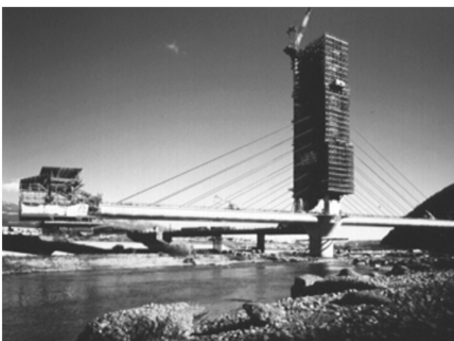
Constructing cable-stayed bridge
