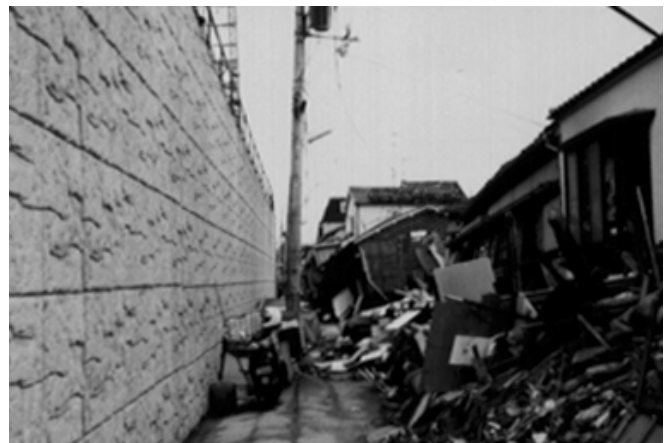
Geosynthetic-reinforced embankment with vertical concrete facing wall undamaged by Great Hanshin Earthquake (RTRI)
