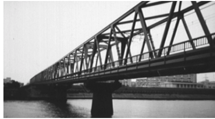
Through truss bridge (RTRI)
