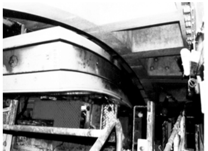
Erecting prefabricated segments behind shield in Tokyo's new Subway Line No. 7 of Teito Rapid Transit Authority (M. Shimizu)
