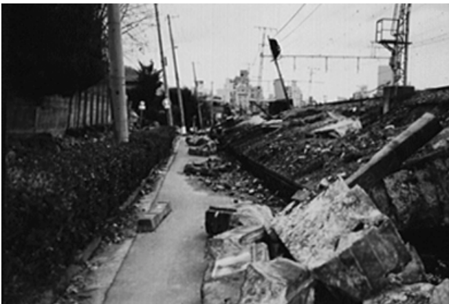
Typical embankment collapsed during Great Hanshin Earthquake (RTRI)
