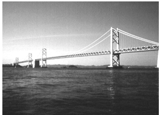
Chain of bridges joining Honshu and Shikoku over Seto Inland Sea—upper deck for motorway and lower deck for railway (Honshu-Shikoku Bridge Authority)
