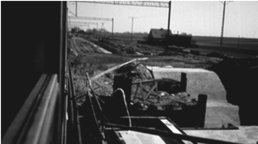
Track improvement works between Warsaw and Poznan
