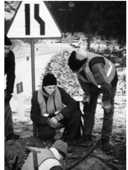
Level crossing work
