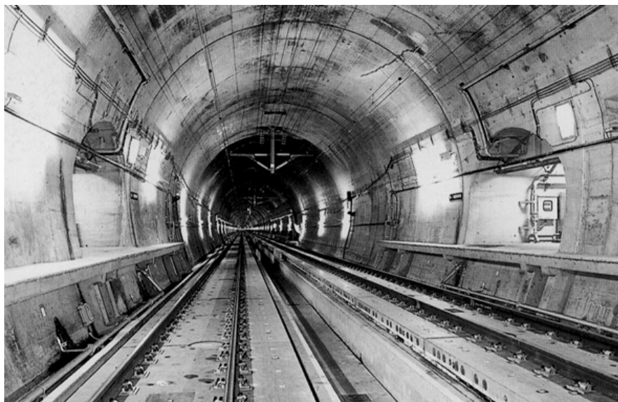
Seikan Tunnel with track bed prepared for eventual shinkansen service (Japan Railway Construction Public Corporation)
