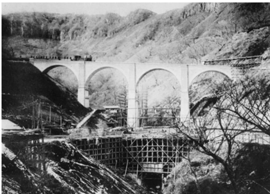
Figure 4 The Usui Viaduct under Construction
