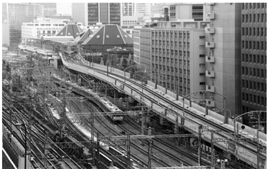
Chuo Line viaduct near Tokyo Central before relocation (top) and after
