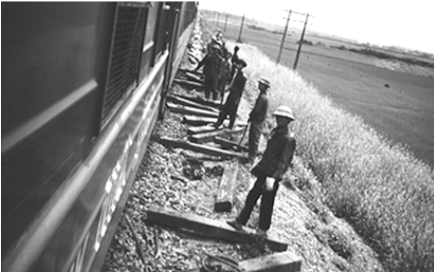
Track workers replacing old sleepers on main line from Hanoi to Ho Chi Minh City in Viet Nam (EJRCE)
