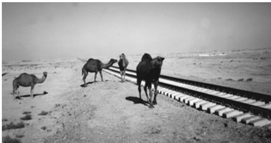
Laying new track across Karakumy Desert (Turkmenistan) to extend northwards
