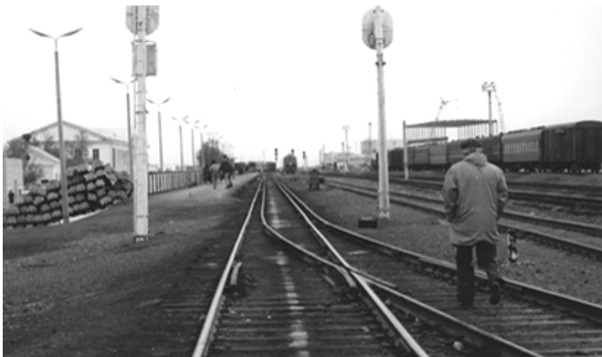
Mixed-gauge (1435/1520 mm) track at Druzhba Station near Kazakhstan–Chinese border
