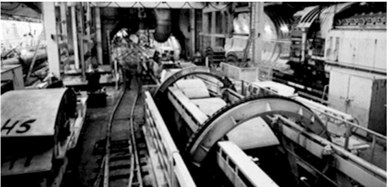
View of two train tunnels and central service tunnel under construction at French side
