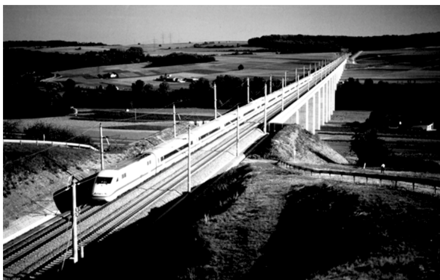
German high-speed ICE at Enztaal Bridge (Mannheim-Stuttgart)
