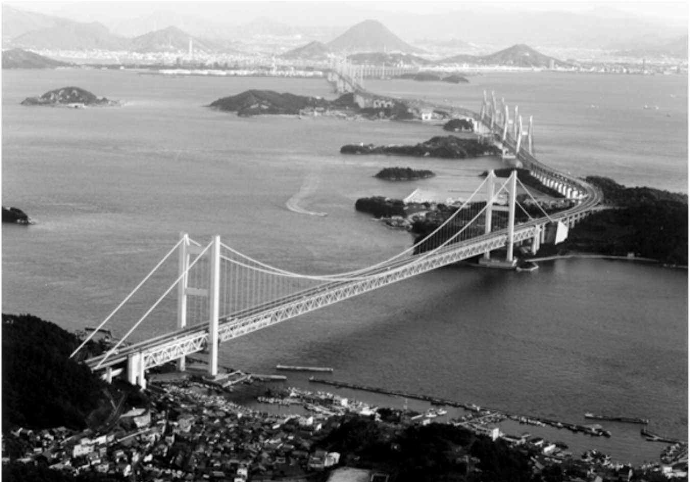
Chain of combined rail and road bridges between Honshu and Shikoku
